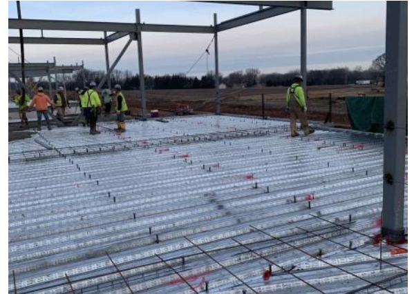
Second floor in classroom wing is prepped for concrete (03/22/2022)
