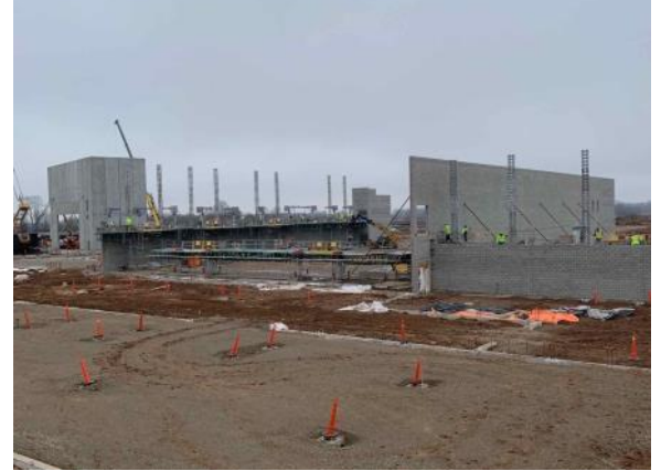
Masonry walls going up in competition gym (03/15/2022)
