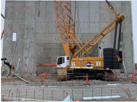
Completion of all 63' tall precast panels in the auditorium (03/17/2022)
