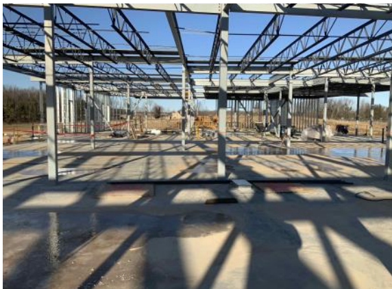
Completed second floor concrete floor (03/28/2022)
