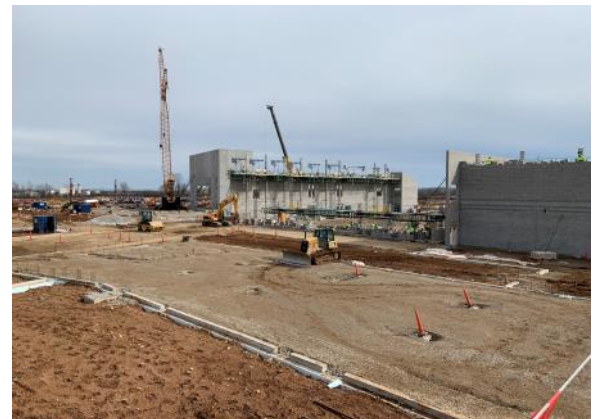
Overview of masonry gym walls and precast walls in the auditorium (03/17/2022)
